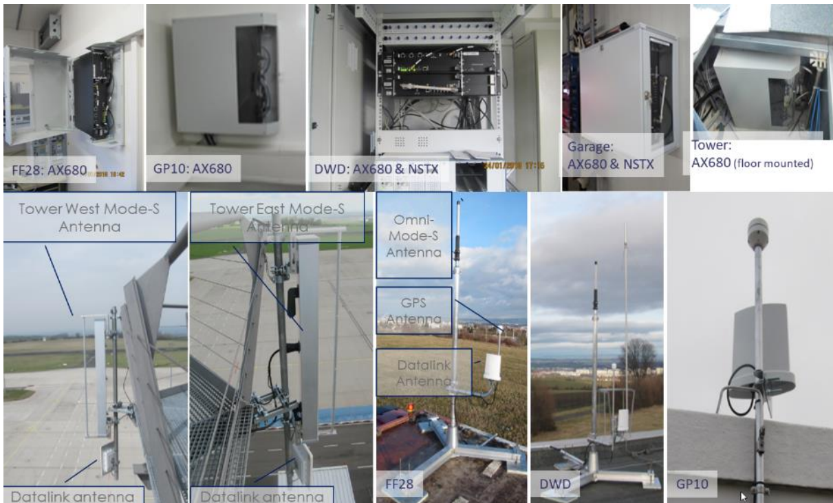
Figure 4-3: Mini-MLAT Equipment used at airport of Erfurt
