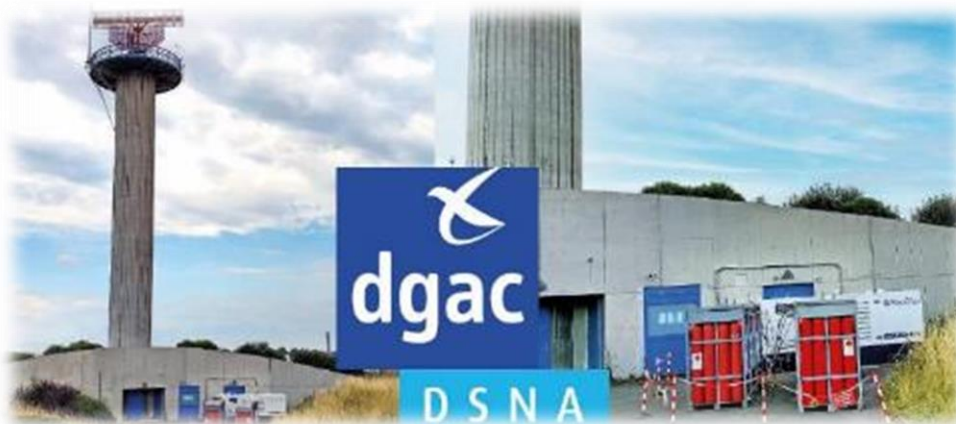
Figure 115: Experimentation #2 – M110 system from POWIDIAN and BOUYGUES Energies & Services
