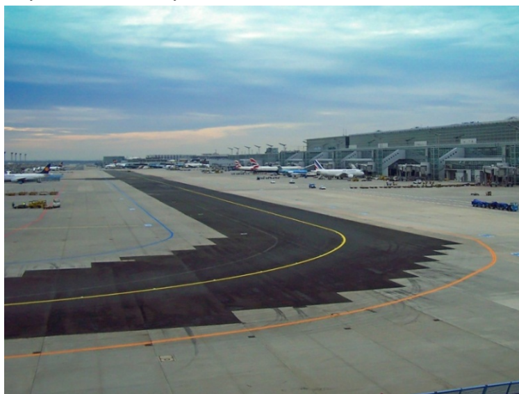
Figure 12: APTR at Frankfurt airport
