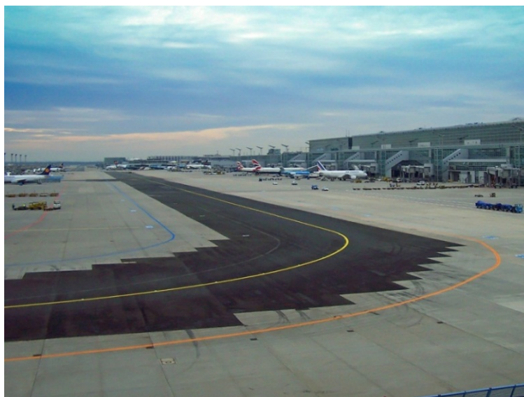
Figure 12: APTR at Frankfurt airport
